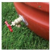
Spread a layer of acrylic caulk around the outside of the spigot for added protection.
