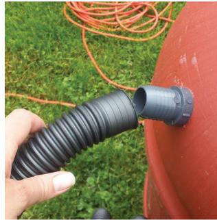
Attach an 8' section of the sump pump hose over the hose barb.
