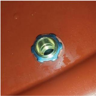
From the inside of the barrel, place the other rubber garden hose washer over the threads of the spigot and tightly screw the locking nut on the threads. (A flashlight may come in handy for this step)
