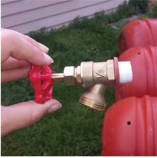
Wrap the spigot with plumber's tape and place a rubber washer flush against the base of the threads.
