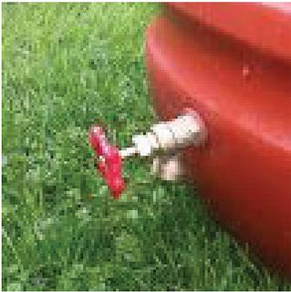
Screw the spigot into the hole until the fitting is snug.
